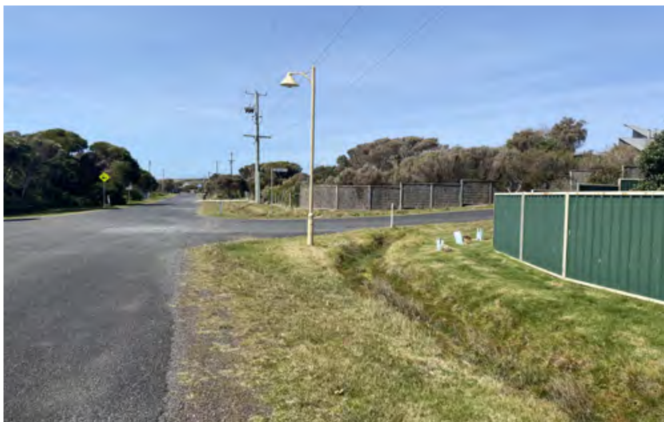
Image: Bellbuoy Beach typical street with open drainage culvert
